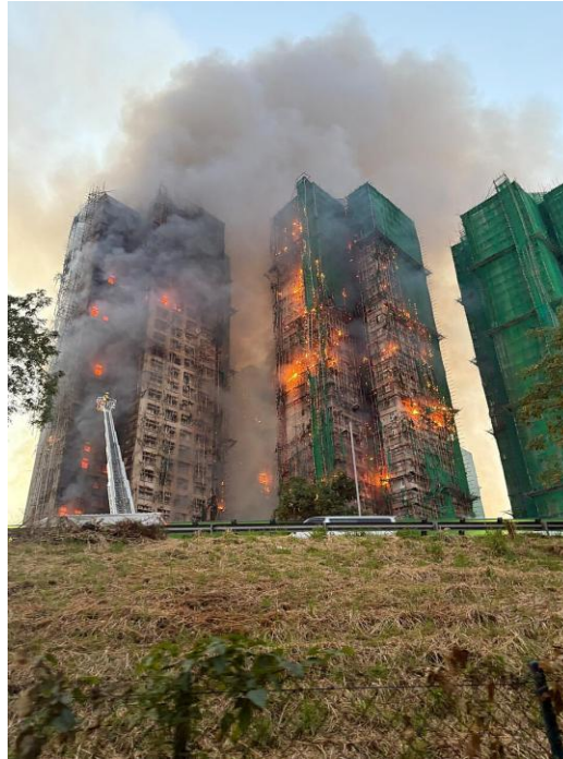
Wang Fuk Court towers on fire, November 26, 2025. Photo: OceanHok, public domain (CC0), via Wikimedia Commons.
