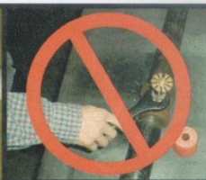
INCORRECT! (sprinkler at floor level)
