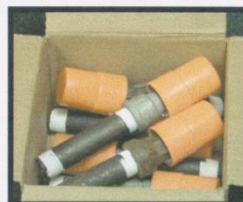
CORRECT (sprinklers protected with caps)
